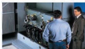
COOPER Power Systems
